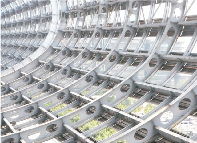
The cold rolled keel welded together to form the shield of train station
